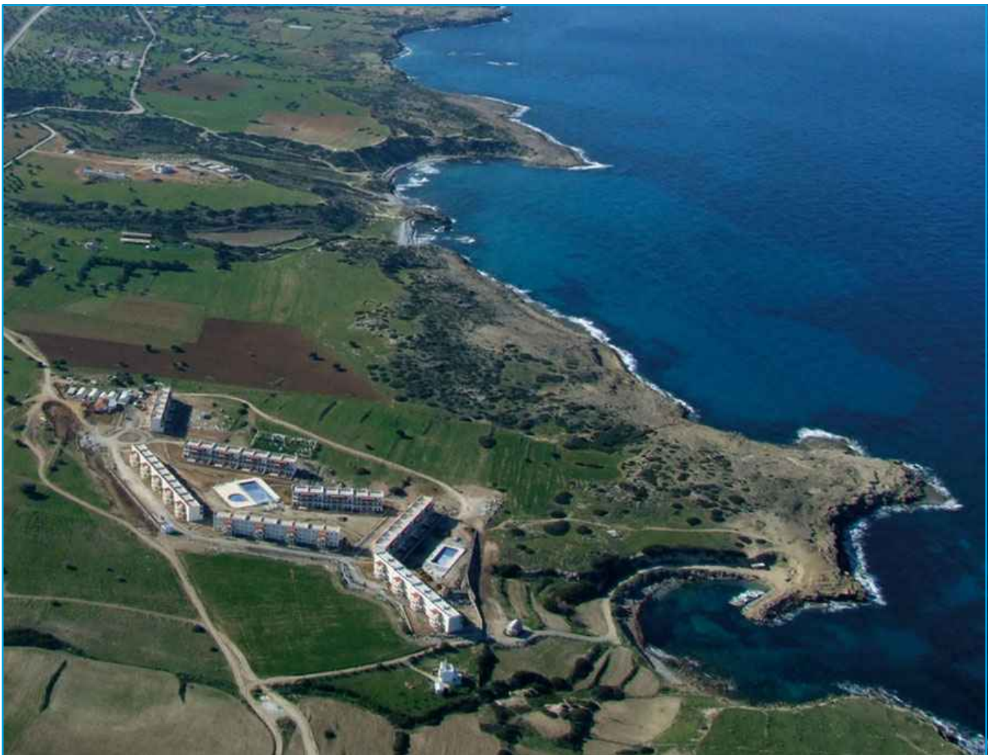
Aerial view - Picture taken during construction
